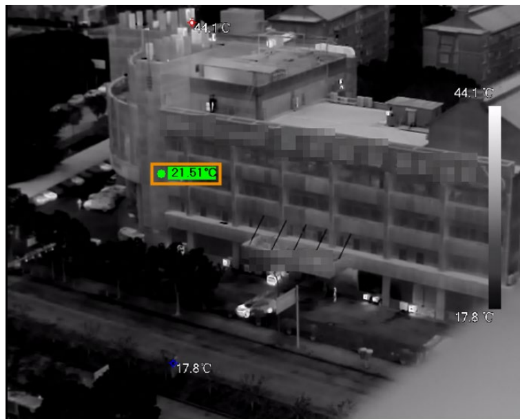
Figure 4-6 Real-time spot temperature measuring
